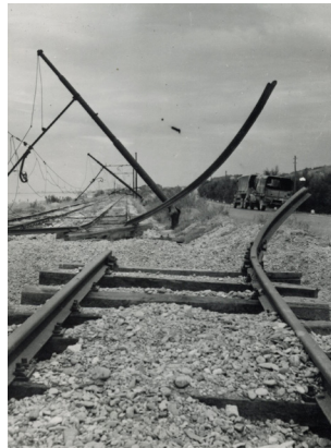
Damaged rail lines, courtesy of 417 Squadron.
